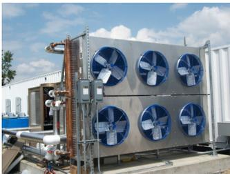
Running parallel to popular air-side Economizers used in commercial air-conditioning, there is a new emerging market for chiller based (or water-side) Economizers. Until recently, deployment of Economizers on chillers have been limited to larger tonnage (150 tons and up) applications mainly due to costs associated with controlling the Economizer systems to deploy at the right time under optimal environmental conditions.
