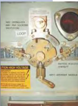
*Anti-reverse handle with provision for locks and switch position contacts*
